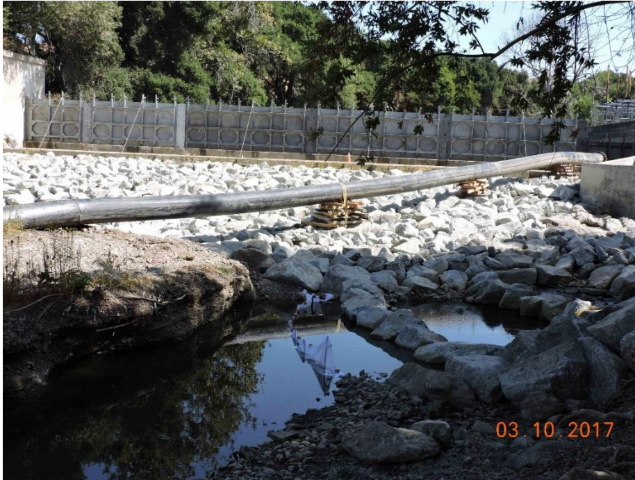
Photo 7. Metcalf Pond dam panels reinstalled and dam apron buttressed with grouted boulders on 3 October 2017. Flow bypassed in pipeline to allow grouted boulder weir construction that was necessitated by channel down-cutting during flood.
