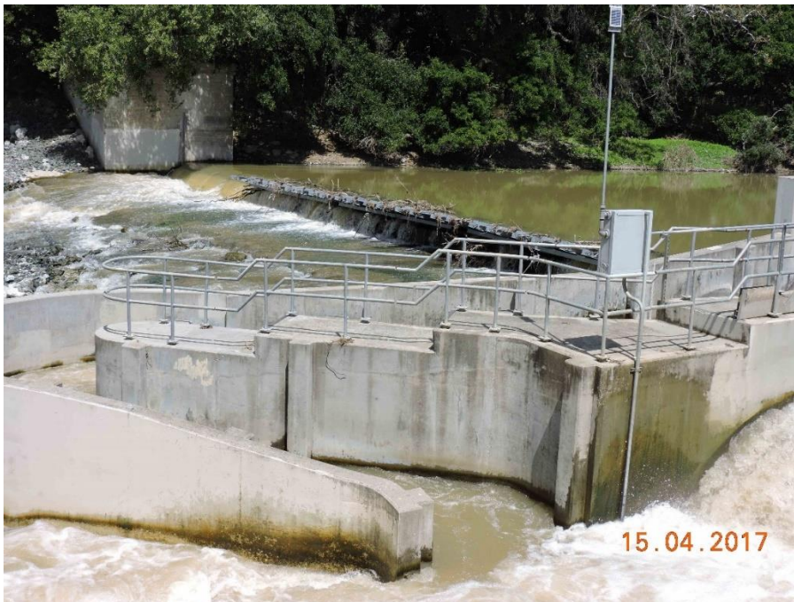
Photo 6. Metcalf Pond Dam on 15 April 2017, with a functioning fish ladder that had been modified for passage by 30 March.
