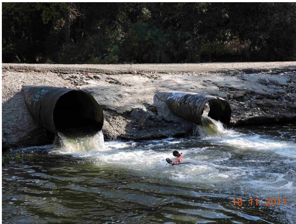
Photo 12. Singleton Road on 18 November 2017 at approximately 50 cfs. Possibly marginally passable through the culverts. Note the damage to culvert on the right in the picture.
