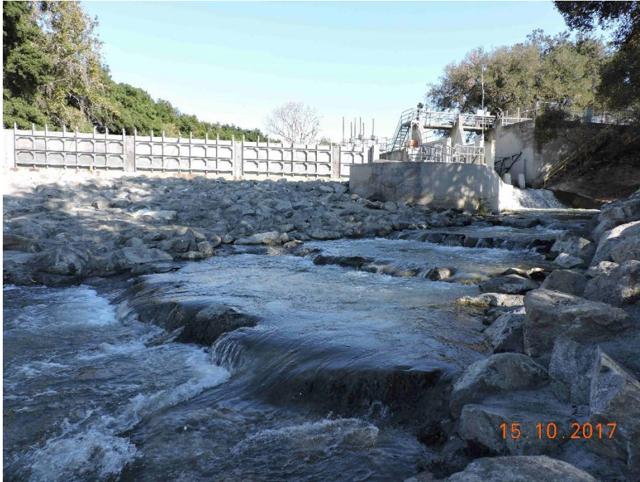
Photo 9. Grouted boulder weirs on 15 October 2017, with pipeline removed and flow through radial gates. Gates were slowly closed (to maintain a live stream downstream) raising the Metcalf Pond water level, and allowing flow to spill through the fish ladder 1 week later.
