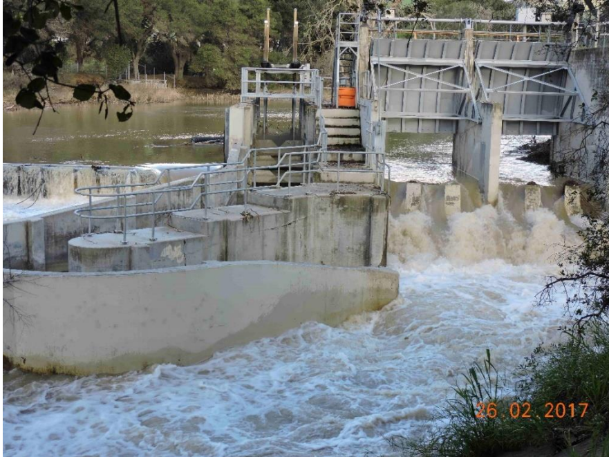
Photo 5. Metcalf Pond radial gates and impassable (no flow) fish ladder on 26 February 2017.
